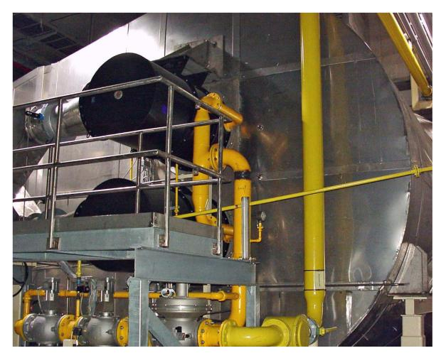
Two gas fired MEGAFIRE® 45M EB burners, total capacity 20 Megawatt heating a recirculating process air stream which feeds a TAD on a paper machine.
